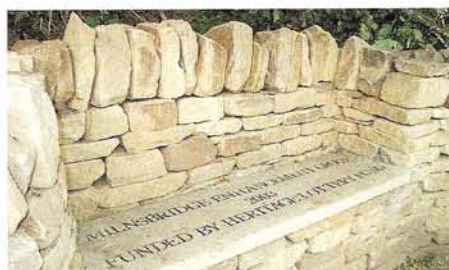
Stone seat built into dry-stone walling at the riverside
